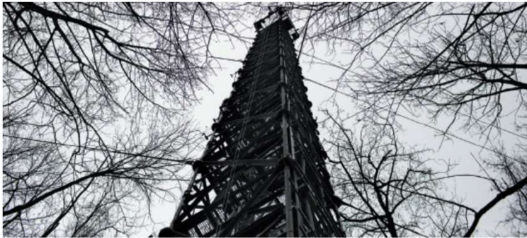
Instruments on a 50-metre-tall tower in western Virginia will monitor the metabolism of the forest by measuring carbon dioxide and water vapour.
